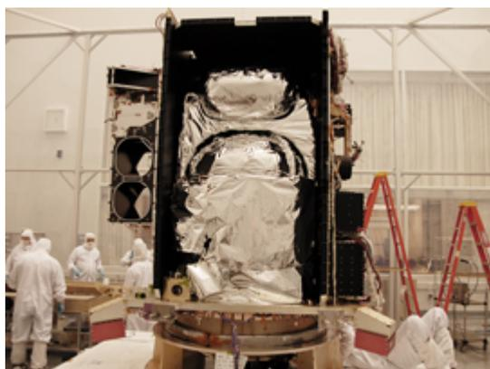
On February 28, 2008, we attached the -Y and -Z panels to the propulsion module, and we also installed the +X panel for stability. This major mechanical operation involved about a dozen engineers and technicians. Since that time, the flight Telemetry, Tracking, and Command unit arrived, and we integrated it with the spacecraft and tested it. On March 1st, the Diviner instrument arrived. We are checking it out this week.
